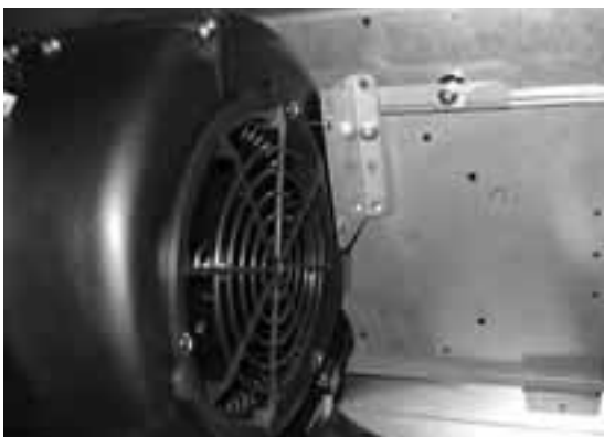
11. Place blower inside round end of round to rectangular transition adapter. Attach blower brackets to blower plate with (4) screws provided.
