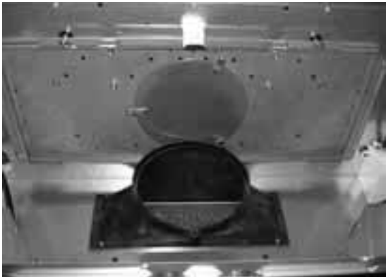
9. Picture of round to rectangular transition adapter installed in hood.
