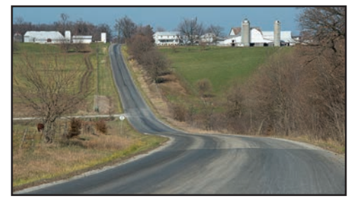
Above: America's rural roads and bridges are in need of repairs and modernization to support economic growth and improve traffic safety in the nation's Heartland, according to a new report released by TRIP, a national transportation non-profit research group (photos courtesy of Joseph L. Murphy, the Iowa Soybean Assoc.)
