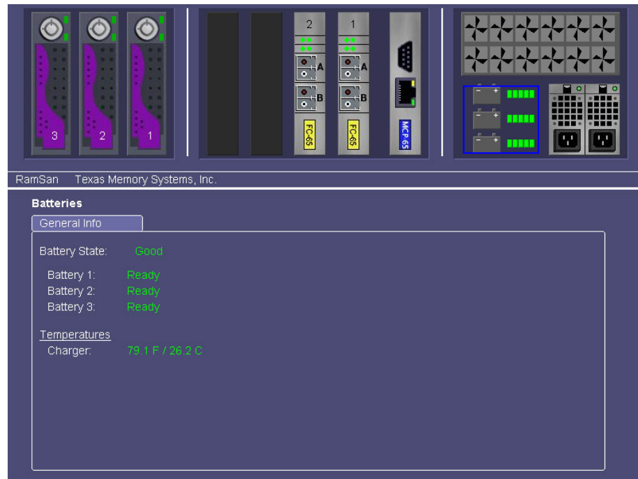
Figure 5-5: Battery Status via Web interface
