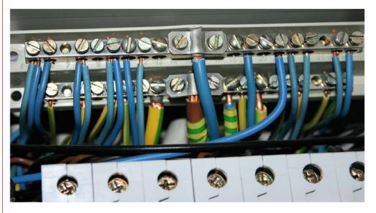
By the way, this is how a proper TN-S installation looks like. Protective and neutral conductors collect on separate equipotential bonding rails – and of course "bridges" are not permitted.
