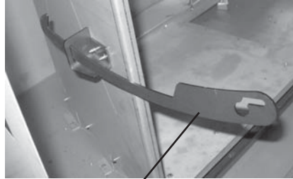
Hinge with door removed.
