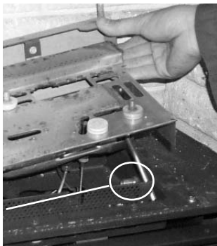
Burner Orifice
