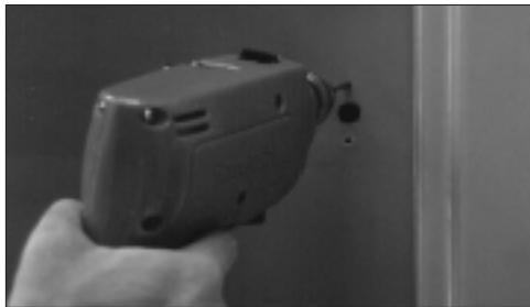
5. Drill holes for mounting backbar and for feeding wires from the loop transfer, per mounting specifications.
