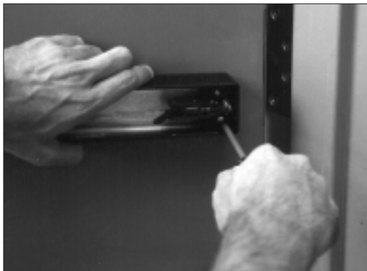
6. Attach wires and mount exit device backbar.
