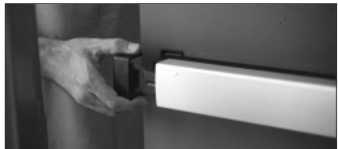
8. Mount end caps to complete pushbar assembly.
