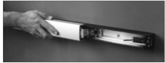
7. Attach pushbar cover by sliding on the right hand scissors first, then back on the left hand scissors until cover seats in position.
