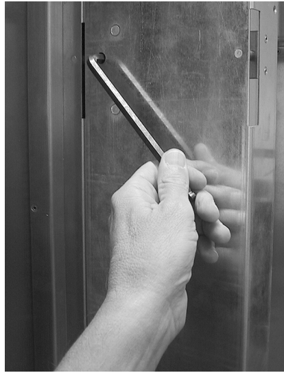
Figure 12. Expansion Bay Installation (c)
