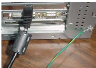
This partial view of the host PC shows the Ethernet cable with a ferrite collar. The PC's connection to the ground-line is also visible.
