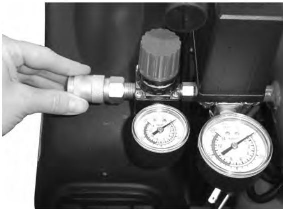
Figure 3. Installing the Air Chuck
