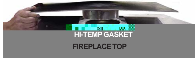
FLUE TILE SUPPORT FOR A MASONRY FIREPLACE
