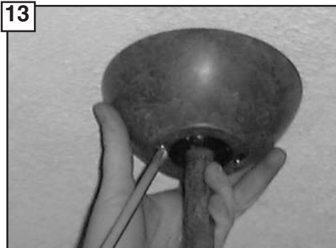
Raise the canopy up and align the two holes in the canopy with the two holes in the hanger bracket. Secure with two screws provided.
