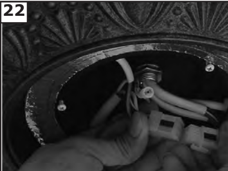
22 Connect plug from fan to switch house plug.
