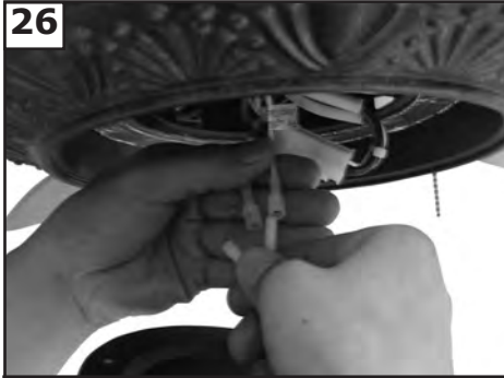
26 Connect white wire from fan to white wire from light fixture. Then plug blue wire from fan to black wire from light fixture.
