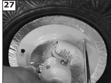
27 Install by twisting clockwise, add 1 screw removed step 23 to light fixture. Tighten the 3 screws securely.
