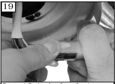
Connect 9 pin plug from fan to switch housing 9 pin plug.
