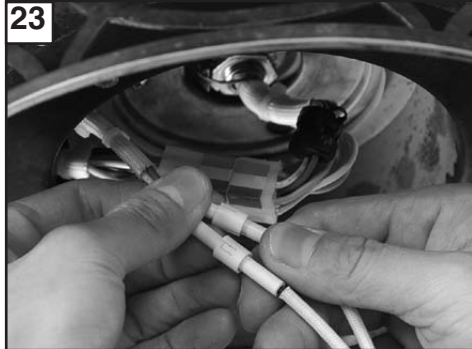
23 Plug white wire from fan to white wire from light kit. Then plug black wire from fan to black wire from light kit.
