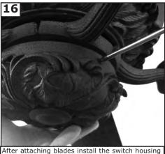
After attaching blades install the switch housing using the three screws previously removed.
