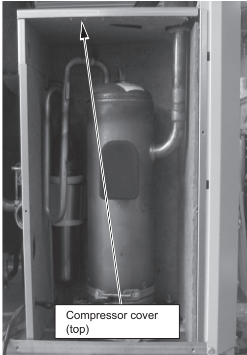
4. Remove the compressor cover (top).
