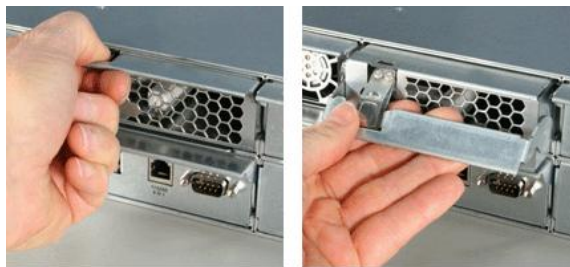
Figure 13: Removing a cooling unit from the enclosure
