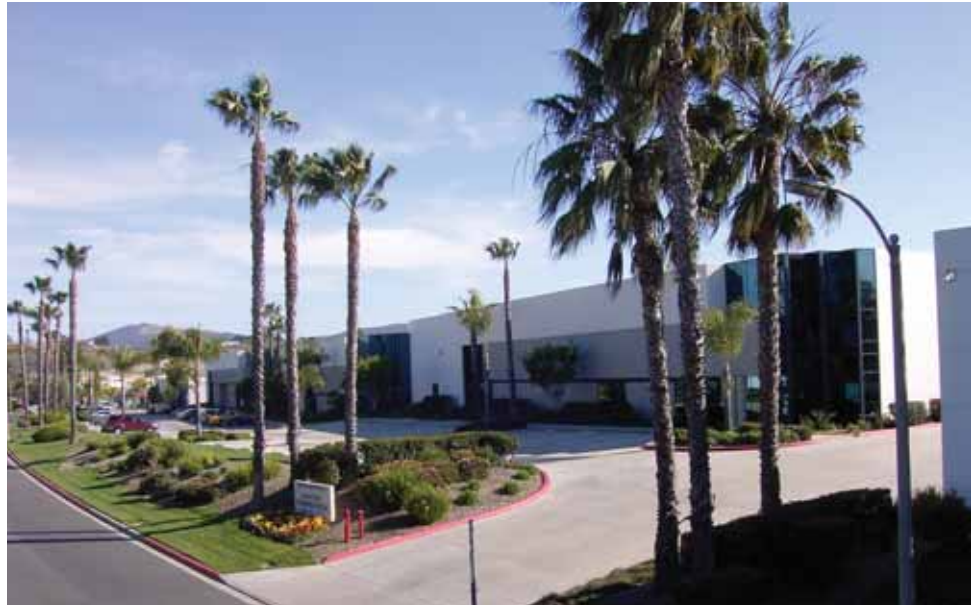
West Coast Distribution Center
