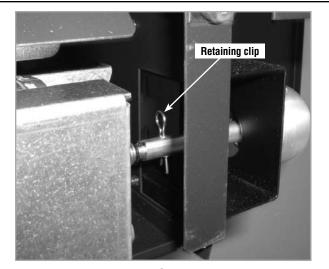
Figure 5 - Remove Retaining Clip
