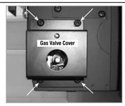
Figure 6 - Remove Gas Valve Cover
