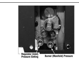
Figure 7 - Manifold and Inlet Pressure Taps
