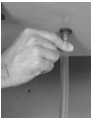
figure 9.2 Insert condensate line
