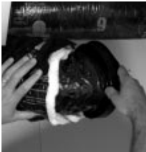
figure 10.2 Insert vinyl duct over the hooks. Fix the collar on the floor joist.
