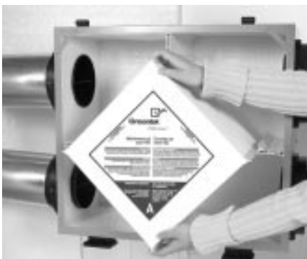
figure 14.3 Slide out the Energy Core
