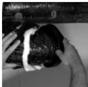
figure 6.2 Insert vinyl duct over the hooks and seal with a 30" Tie wrap.
