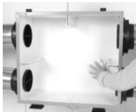
figure 14.4 Wash the Walls of the Unit
