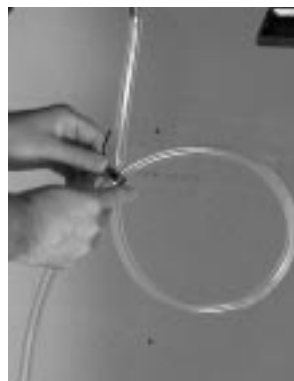
figure 9.3 Make a loop in condensate line
