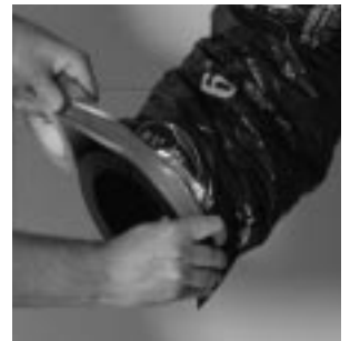
figure 10.4 Finish by taping the duct on the collar.
