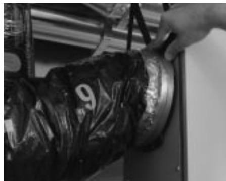
figure 6.5 Slide collar on the unit.
