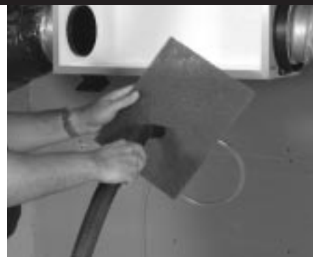
figure 14.2 Vacuum the Filters
