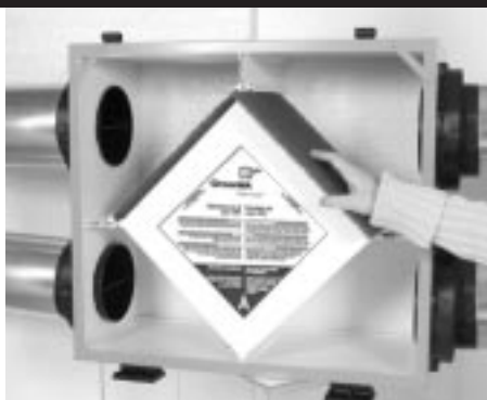
figure 14.1 Slide Out the Filters
