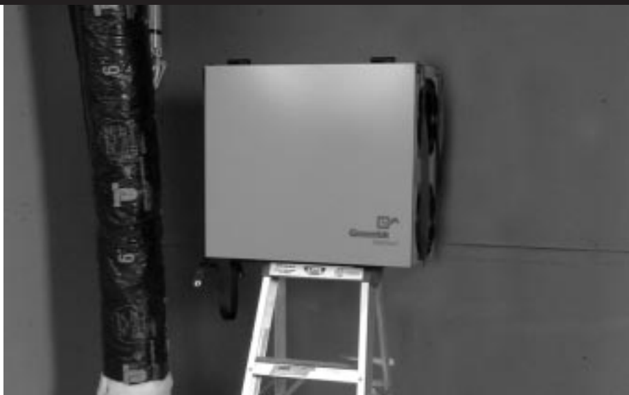
figure 5.1 Place HRV on a stepladder
