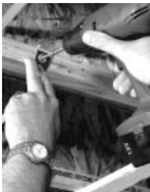
figure 5.2 Attach your four straps to the floor joist making sure that you attach thru the grommets.
