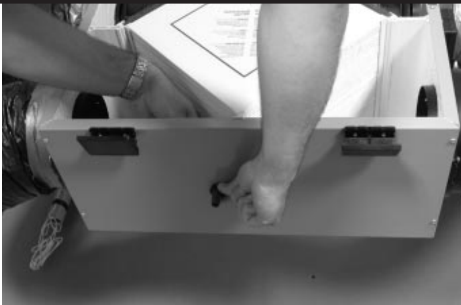
figure 9.1 Hand screw the drain adapter
