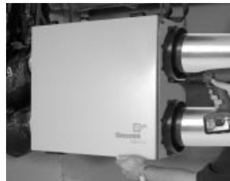
figure 6.6 Fix and secure with four screws supplied.
