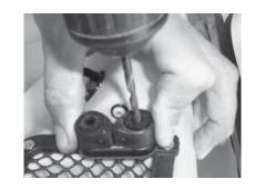
19. Place the padeye fitting over the cleat. Using the provided hardware, through bolt the cleat to the kayak. You will need to reach inside of the middle hatch to put on the washers and nuts on the inside of the kayak.
