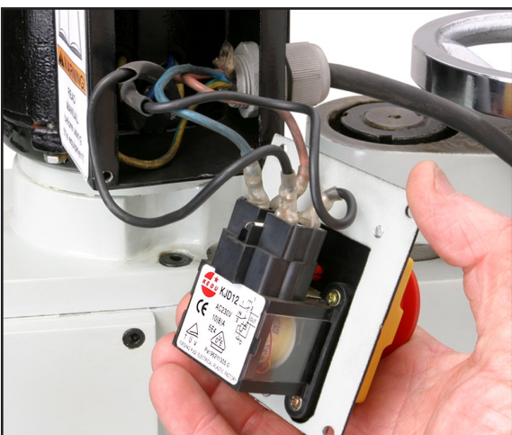
Figure 66. Mill power switch.
