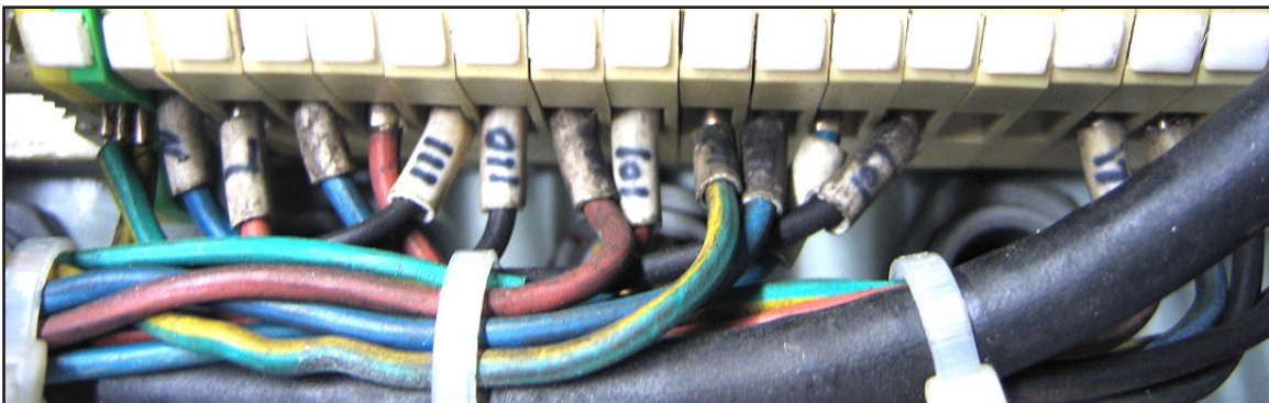
Figure 63. Junction block wiring.
