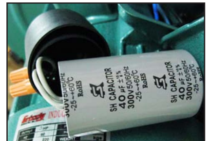
Figure 61. Run capacitor.
