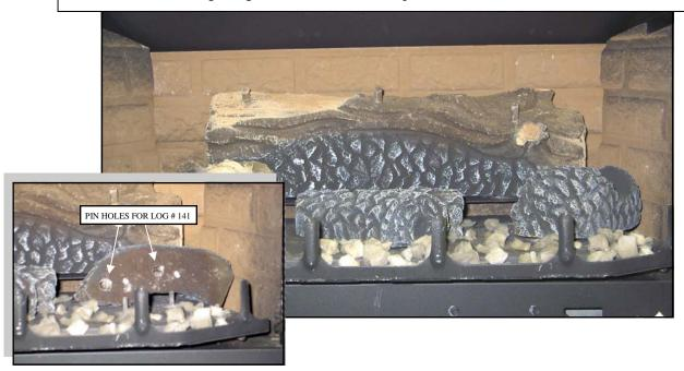
**STEP 6** - Locate log #135 and place onto rear log using the locator pins and pre-drilled holes in log. Log should sit as shown in photo below.
