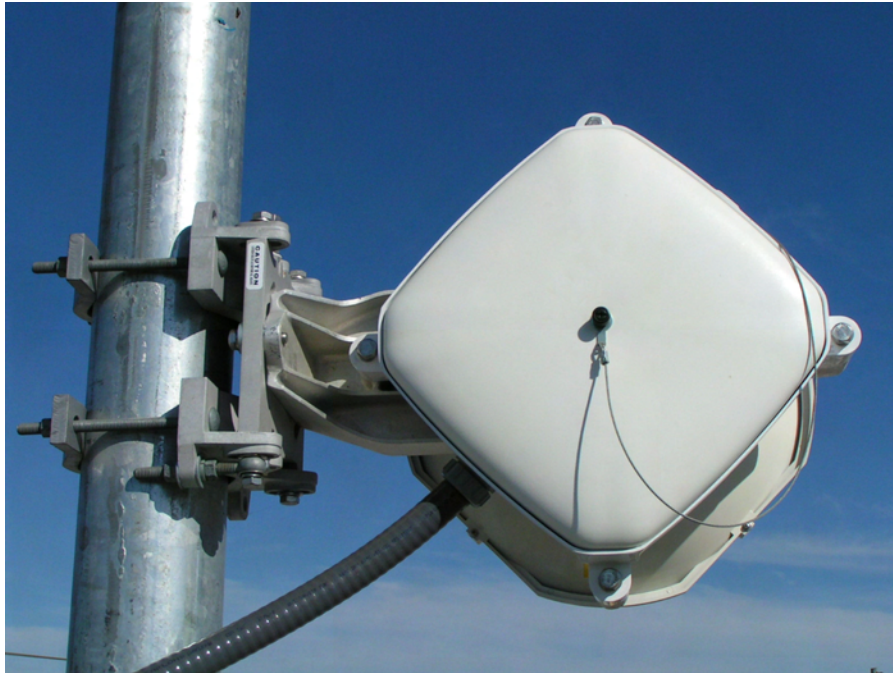
Figure 3-11: Back view of fiber and power cable installed on a vertically polarized unit. Notice that the cable conduit is on the left hand side when the radio is in (V) polarization.
