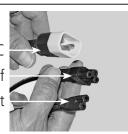
**Step 4:** Connect an IEC connector into the top IEC power strip. Continue this action until all 16 IEC leads are connected.
