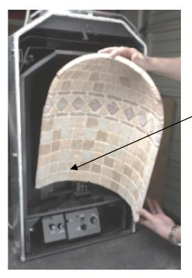
(a) Tilt the liner forward and at a slight angle as you insert it into the firebox.
