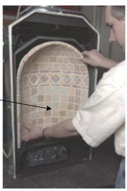
4 Replace the burner, logs, embers, glass and face.
