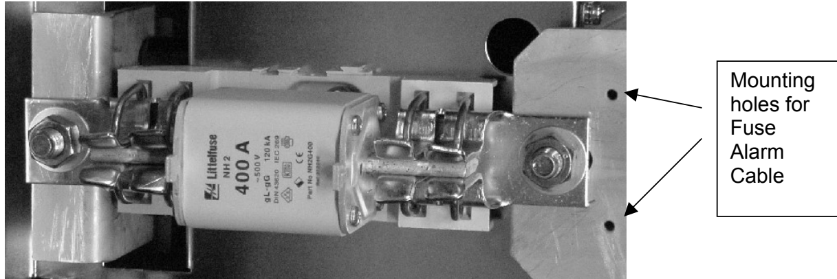
Figure 3.7-6 NH2 Fuse Connections
