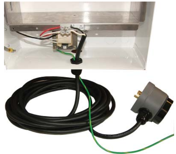
Fig. 4-4, Streetlight AC Power Tap Cable Installed
