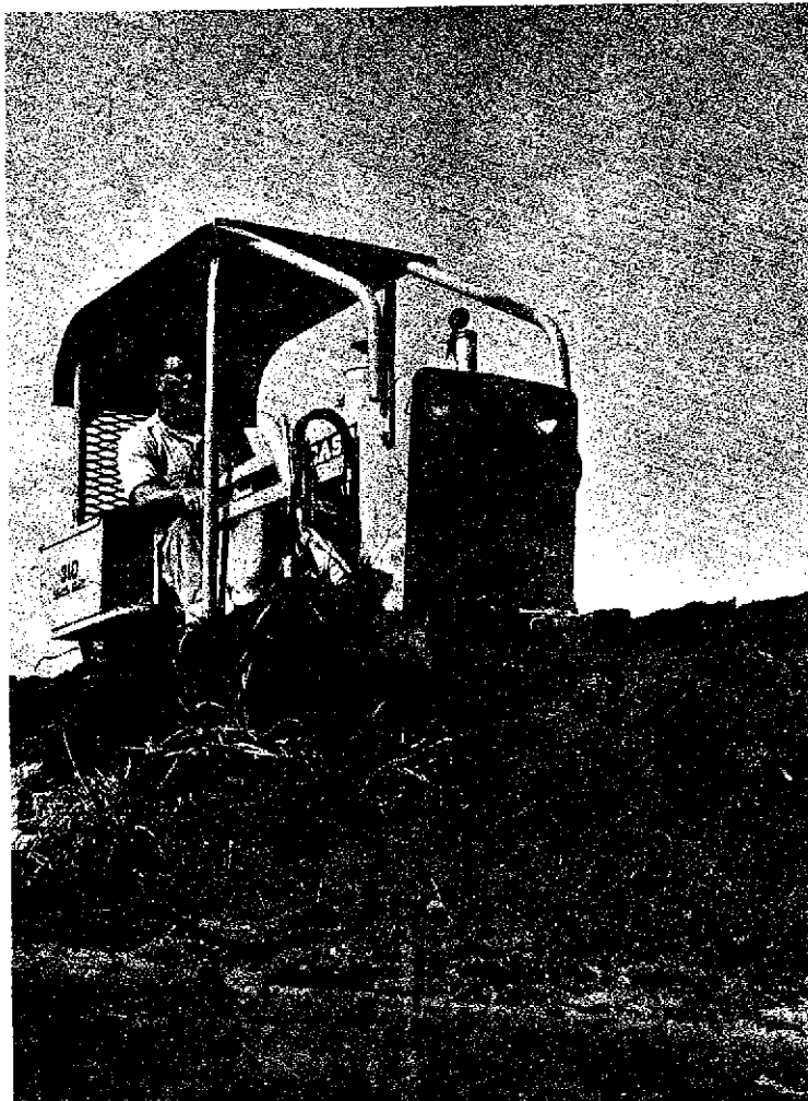
GROUND WAS broken Tuesday for the first dam at the Callahan Mining Corporation site on Cape Rosier. At the bulldozer controls is Lloyd Fowler, Brooksville.--Packet photo.
